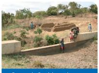
3R example: Sand dams, these are small scale dams that capture sediment and water during the wet season, thus creating groundwater storage in the newly created aquifer behind the dam.
